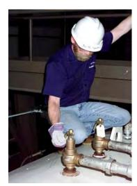
Avoid excessive operation of the safety valve; even one opening can provide a means of leakage. Safety valves should be operated only often enough to assure that they are in good working order. When a pop test is required, raise the operating pressure to the set pressure of the safety valve, allowing it to open and reseat as it would in normal service.
