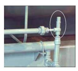
Oil pressure is regulated at several points. The first is at the relief valve at the oil heater. The relief valve should be set so that at maximum firing rate a minimum reading of 75 psi is obtained on the oil supply pressure gauge.
