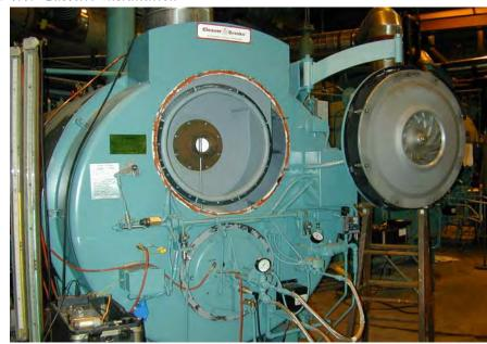
FIGURE 8-23. Fan/Motor Cassette Open
