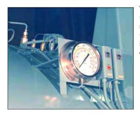
The dial settings are generally accurate, although it is not unusual to have a slight variation between a scale setting and an actual pressure gauge or thermometer reading. Always adjust control settings to agree with pressure gauge or thermometer readings. Accurate instrument readings are required. When necessary use auxiliary test equipment to set controls.
