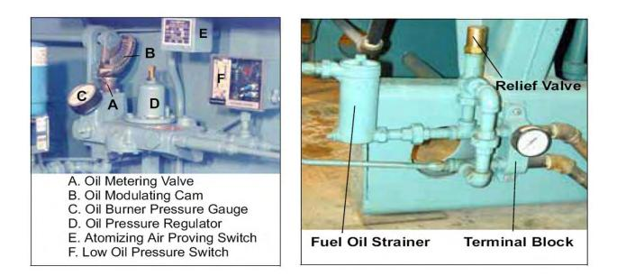
FIGURE 2-9. Fuel Oil Controller and Relief Valve & Terminal Block
