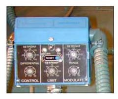
Turn the adjusting screw until the indicator is opposite the low point of the desired modulating range. Modulated firing will range between the low point and a higher point equal to the modulating range of the particular control. In 0-15 psi controls the range is 1/2 lb; in 5-150 psi controls the range is 5 lbs; in 10-300 psi controls the range is 12 lbs.
