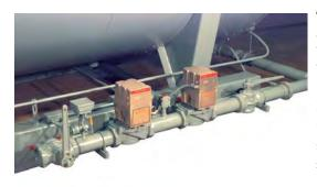
The motorized gas valve (Hydramotor) operating mechanism is completely immersed in oil and little maintenance is required because of the sealed design. However, proper operation should be checked on a routine periodic basis.
