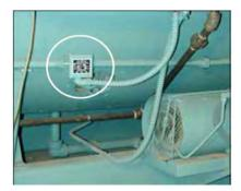
The air pressure against the diaphragm actuates the switch which, when closed, completes a circuit to prove the presence of atomizing air. Since the pressure of the atomizing air is at its minimum value when there is no fuel present at the nozzle, adjustment of the switch should be done while the unit is running but not firing. The control should be set slightly below the minimum pressure, but not too close to that point to cause nuisance shutdowns.
