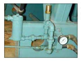
Oil supply pressure is regulated by adjusting the pressure relief valve at the oil terminal block. A pressure gauge should be installed in the terminal block and the relief valve adjusted to obtain a minimum reading of 75 psi when the burner is firing at maximum rate.
