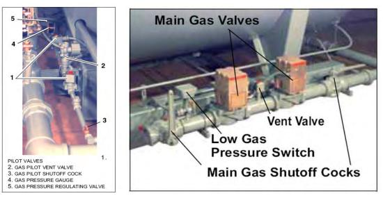
FIGURE 2-6. Pilot Gas Train and Main Gas Train
