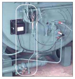
FIGURE 2-7. Burner Drawer Face and Gas Modulating Cam
