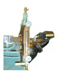
Always be sure of the boiler water level. On steam boilers, the water column should be blown down daily. Check samples of boiler water and condensate in accordance with procedures recommended by your local Cleaver-Brooks authorized representative. Refer to Sections 3.7 and 3.8 for blowdown instructions and internal inspection procedures.
