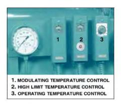
FIGURE 6-8. Hot Water Controls
