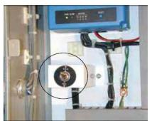
Burners equipped to burn oil and gas (combination burners) include equipment for each distinct fuel. Since the burner uses only one type of fuel at a time, a gas/oil selector switch is incorporated.
