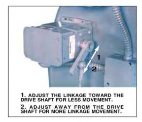
The modulating motor has a 90° shaft rotation. The motor manufacturer also provides a 160° stroke model for other applications. If a replacement is obtained from someone other than a Cleaver-Brooks Service or Parts representative, it may have an incorrect stroke. To prevent damage, determine the 90° stroke prior to installing a replacement.
