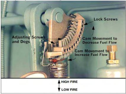
FIGURE 6-13. Fuel Modulating Cam
