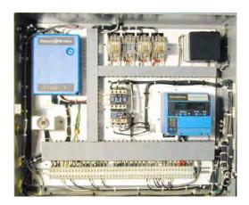
Your spare control should be stored in a dry atmosphere and wrapped in plastic. During an extended shutdown (e.g., seasonal), the active control should be removed and stored. Moisture can cause problems with control operation.
