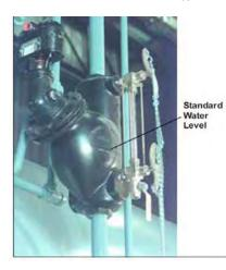
No adjustment is required since LWCO controls are preset by the original manufacturer. However, if the water level is not maintained, inspect the devices immediately and replace as required.
