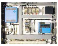
Gas-Oil Switch: Burners equipped to burn either oil or gas include equipment for each fuel. The selector switch engages the appropriate interlocks and controls for gas or oil operation. Chapter 4 details the required mechanical functions of each fuel system.
