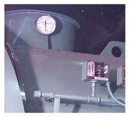
**FIGURE 8-1. Stack Thermometer**
