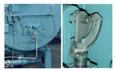
Inspection of the air damper and linkage bearings should be performed on a more frequent basis if the boiler is operating in a dirty environment.
