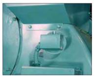
Air pressure against the diaphragm actuates the switch which, when made, completes a circuit to prove the presence of combustion air. since the pressure of the combustion air is at its minimum value when the damper is full open, the switch should be adjusted under that situation. It should be set slightly below the minimum pressure, but not too close to that point to cause nuisance shutdowns.
