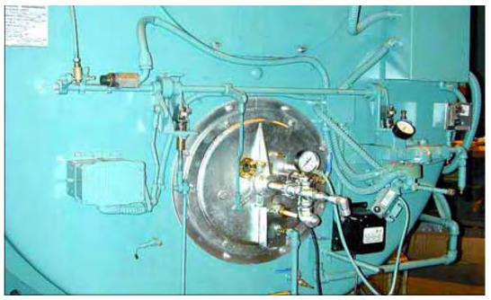
FIGURE 2-19. Burner Drawer and Fuel Linkage Assembly
