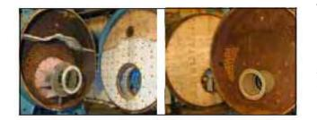
The front door and rear door provide the seal to contain the hot combustion gases. Baffles designed into the doors serve to redirect the combustion gases through the various firetube passages. The flame originates in the furnace. As the combustion gases travel down the furnace and through the various firetube channels, heat from the flame and combustion gases is transferred to the water.
