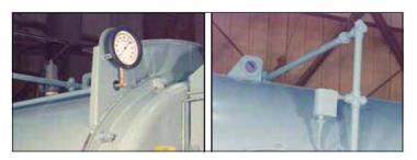
**1.Steam Pressure Gauge**: Indicates boiler internal pressure.
