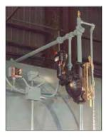
**1.Water Column Assembly**: Houses the low water cutoff and pump control and includes the water gauge glass and shutoff cocks.
