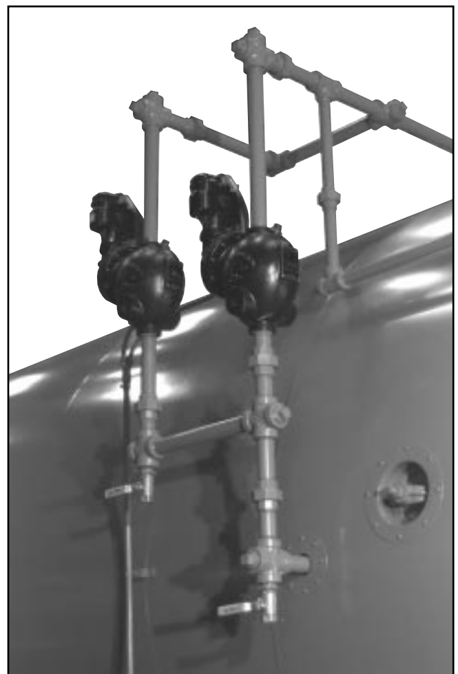
Figure: 1-8 Auxiliary Low Water Cut Off
