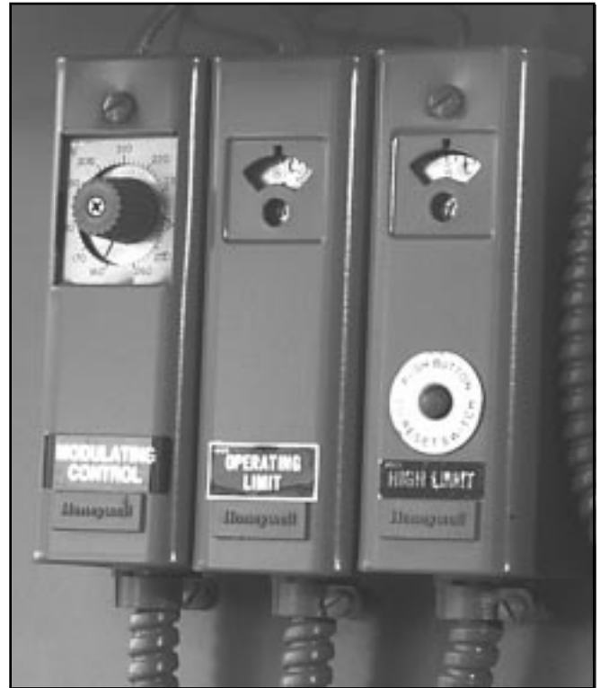
Figure: 1-12 Hot Water Controls
