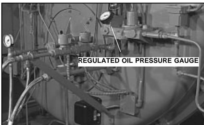
Figure: 5-8 Oil Piping
