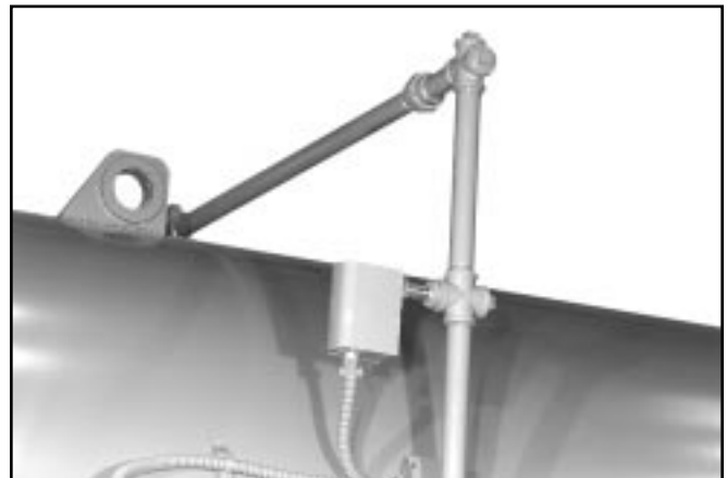
Figure: 1-13 Low Water Cutoff (LWCO Hot Water)
