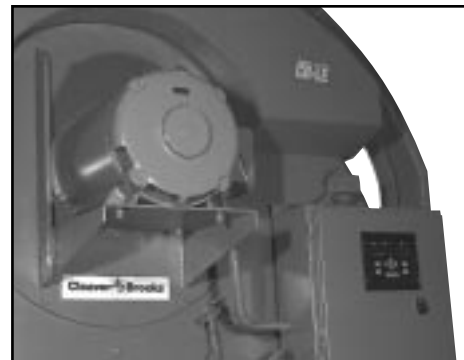
Figure: 2-7 Forced Draft Fan Motor CB-LE
