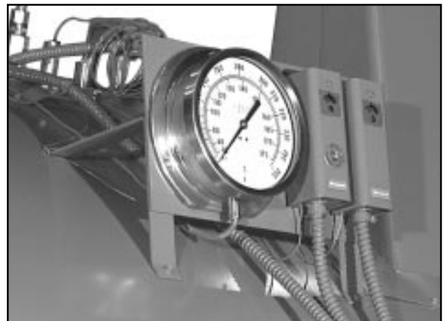
Figure: 6-5 Hot Water Controls
