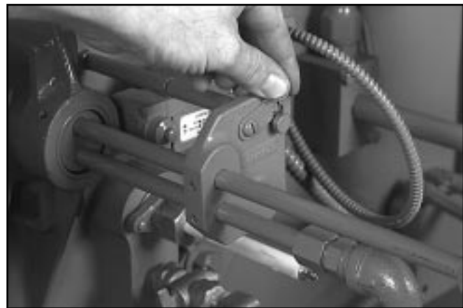
Figure: 6-18 Oil Gun Locked Out
