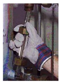
It is recommended that the boiler is off and cool when the glass is replaced.
