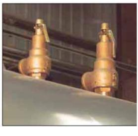
FIGURE 1-4. Safety Valve Piping and Safety Valves
