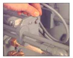
•If the burner is a combination fuel model, set the gas/oil switch to "gas." Withdraw the oil burner gun and latch it in its rearward (lockout) position.
