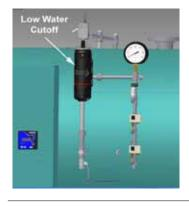
No adjustment is required since LWCO controls are preset. However, if the water level is not maintained, inspect the devices immediately and replace as required.
