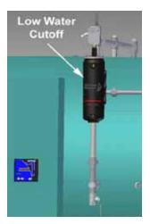
Always be sure of the boiler water level. On steam boilers, the water column should be blown down daily. Check samples of boiler water and condensate in accordance with procedures recommended by your local Cleaver-Brooks authorized representative. Refer to Chapter 3 for blowdown instructions.
