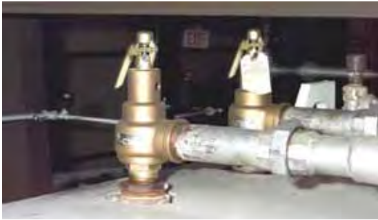
FIGURE 8-4. Safety Valves
