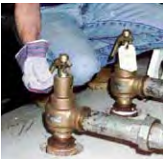
FIGURE 8-5. Operating Safety Valves
