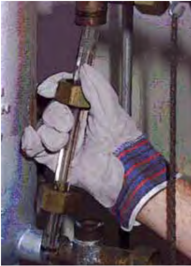
FIGURE 8-3. Water Column Gauge Glass Replacement
