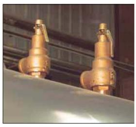
FIGURE 1-4. Safety Valve Piping and Safety Valves
