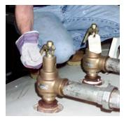
Avoid excessive operation of the safety valve; even one opening can provide a means of leakage. Safety valves should be operated only often enough to assure that they are in good working order. When a pop test is required, raise the operating pressure to the set pressure of the safety valve, allowing it to open and re-seat as it would in normal service.
