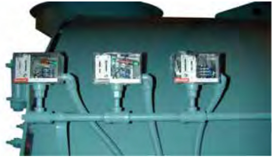
Figure 4-5: Steam Operating Controls
