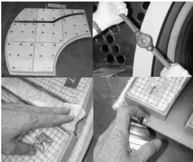
Figure: 5-10 Prepare Doors for Closing and Sealing
