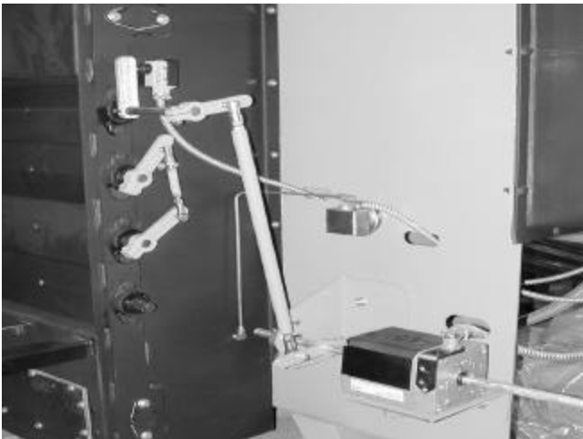
Figure: 5-6 Damper Linkage
