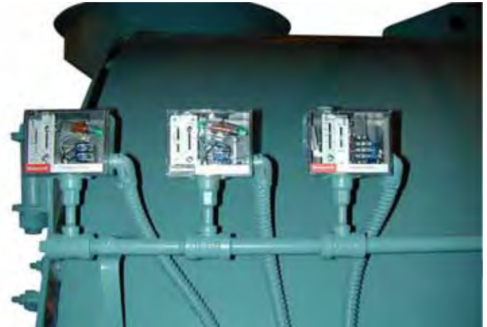
Figure 4-2: Steam Operating Controls
