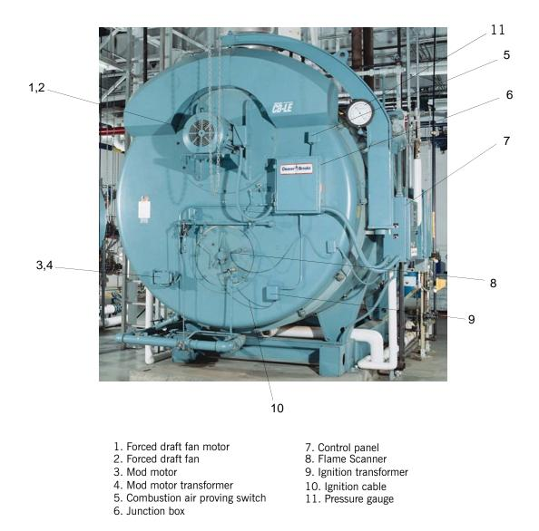
Figure 2-2 Controls/Components Common to All Boilers
