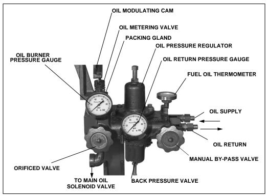
Figure 2-12 Oil Control Valve Assembly - Heavy Oil
