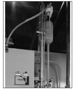
Figure 1-4 CB Level Master (CB-LE high pressure steam)
