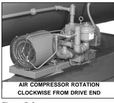
Figure 5-2 Air Compressor CB-LE (CB Option)
