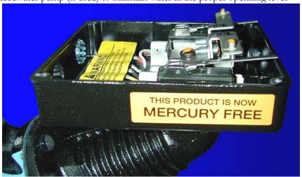
FIGURE 1-4. Low Water Cutoff Pump Control.
