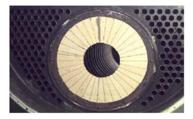
FIGURE 8-13. Refractory Throat Tile
