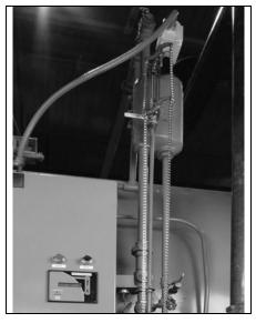
Figure 1-4 CB Level Master (CB-LE high pressure steam)
