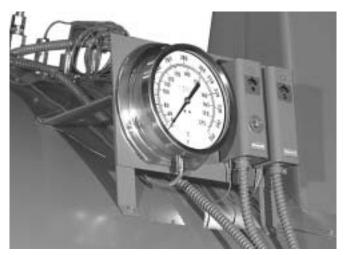
Figure 1-10: Water Temperature Gauge
