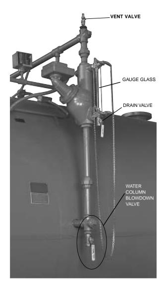
Figure 1-5: Water Column Assembly
