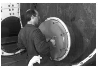
Figure: 8-7 Removing Rear Access Plug
