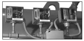
Figure 6-5: Steam Operating Controls
