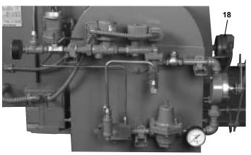
18. COMBUSTION AIR PROVING SWITCH Figure 2-5: Combustion Air Proving Switch 750-179
