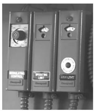
Figure 1-11: Water Temperature Controls
