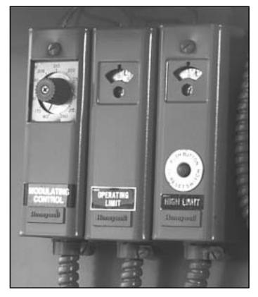
Figure 6-3: Hot Water Operating Controls
