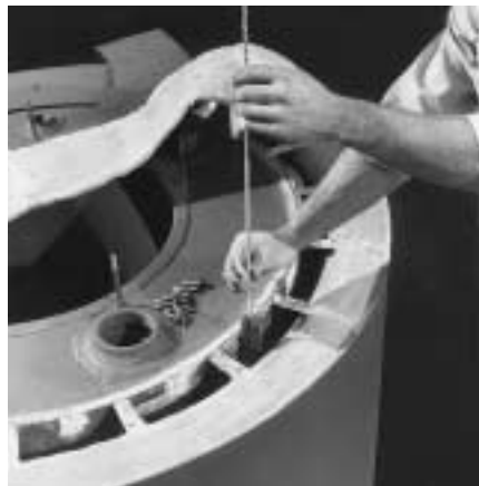
Wire brushing the flue passages.
