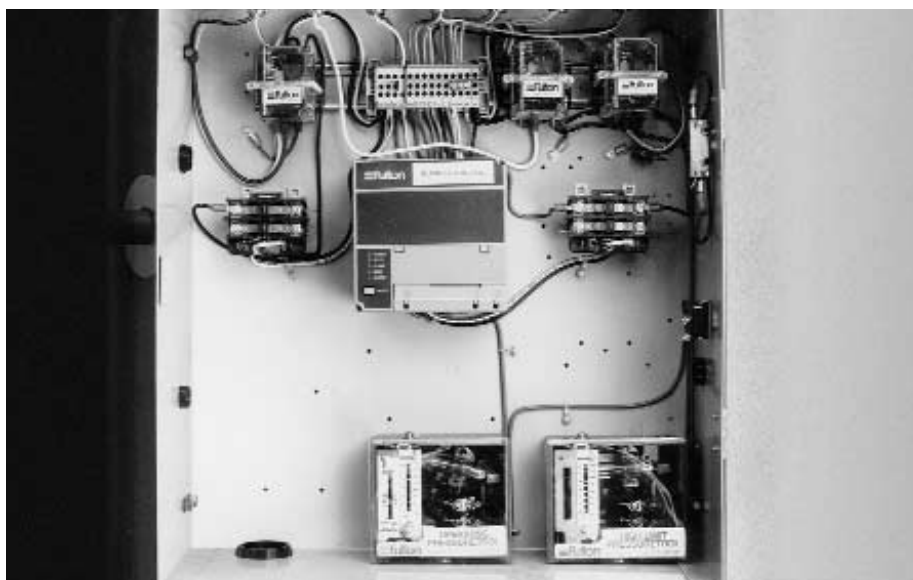
4-50 HP – 7895 flame safeguard control
