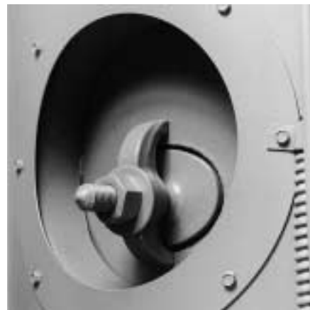
Inspect hand holes for scale or sludge buildup.
