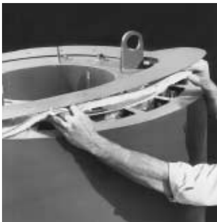
Remove burner and flue cover plate
