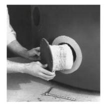
FIGURE 9 - REMOVING CLEAN OUT PLUGS
