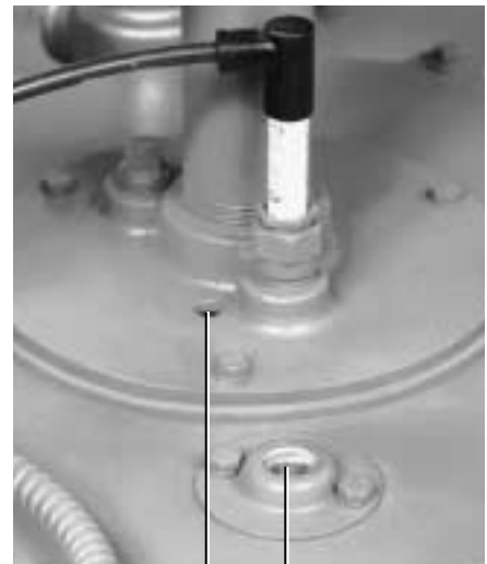
Burner Viewing Port
