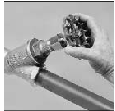
Blow Down Boiler Daily. Shown is the blow down "Y" valve.
