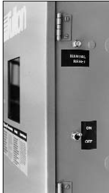
7. Activate the boiler power on switch, located on the side of the panel box.
