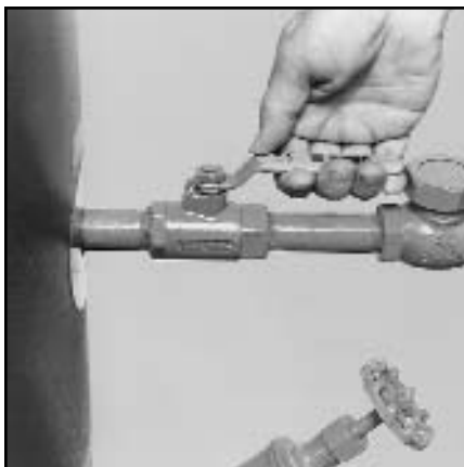
5. Open valves on makeup water line to return if return system is used.
