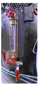
for approximately five seconds, then close the valves. On boilers with float type level devices, refer to the water column cut sheet for proper blowdown technique. Any water column on the system should be blown down daily following the above processes.
