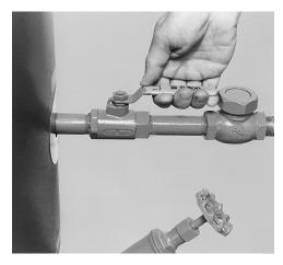
5. Open valve on makeup water line to return, if return system is used.
