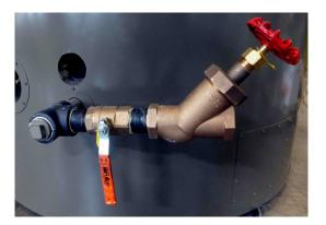
2. Blow down water column each morning when boiler is at 10 PSI (.703 kg/cm2) by opening the water column and the water gauge blowoff valves
