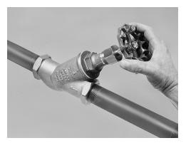
2. Close water gauge drain valve.
