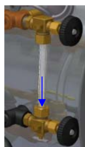
Slide glass up, pull out on bottom of glass and remove.
