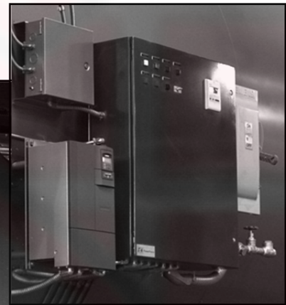
Example of multiple junction box's including: Burner control panel, power disconnect, VFD controller, and junction box, Figure 31c
