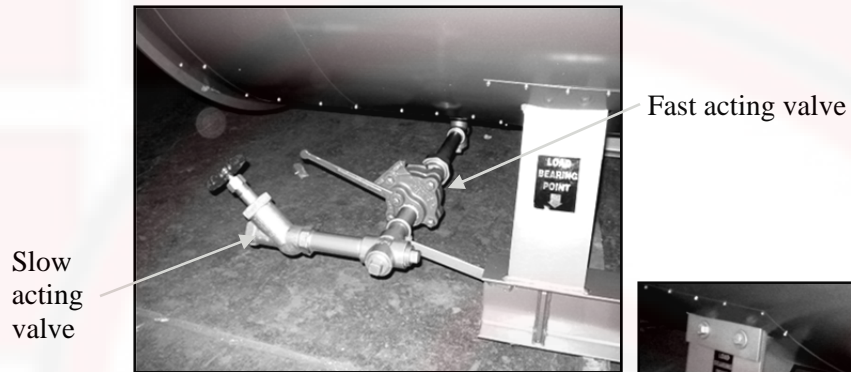
Blowdown valves, single connection: Figure 33
