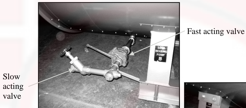
Blowdown valves, single connection: Figure 27
