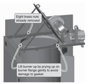
Figure 79 Burner removal and replacement
