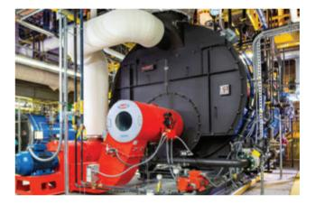
Low NOx by flue gas recirculation can be achieved by one of two methods either forced FGR or induced FGR, depending on application. Forced FGR is accomplished by forcing the flue gases with a separate fan back into the combustion zone. Induced FGR draws the flue gases through the combustion air fan. Both
