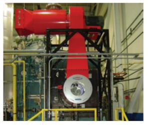
Installation arrangements are limitless. However, for arrangements not shown please contact the factory for consultation in proper air duct design. It is recommended that the pressure drop in the air duct between the outlet of the blower and inlet to the burner be no more than  $\frac{1}{2}$ " WC.
