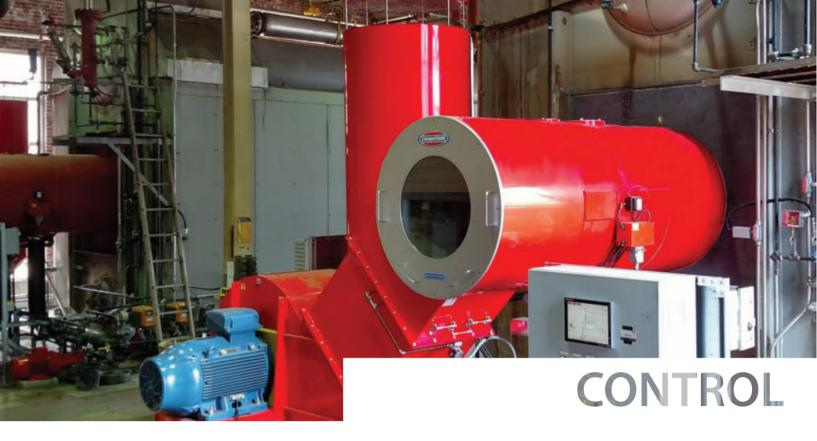
Limpsfield Combustion offers its users control panels to accompany the burners. These are designed and built around advanced combustion control equipment which will further enhance the reliability and performance of the LC burner.
