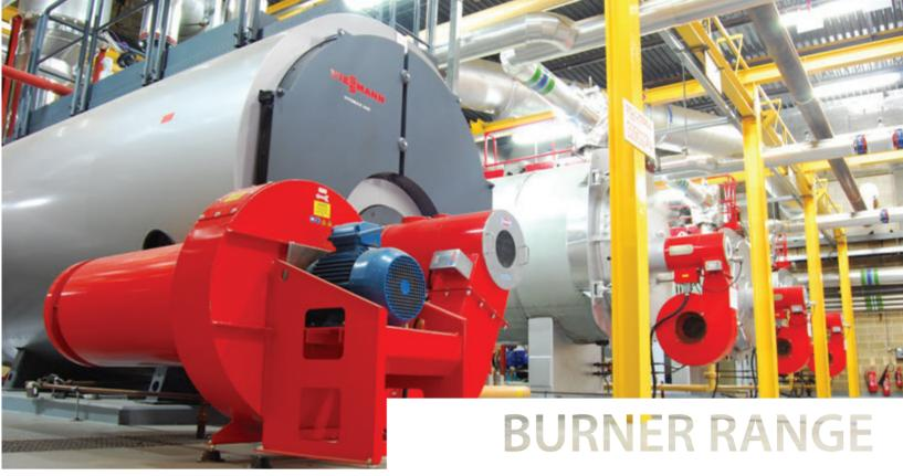
Limpsfield Combustion offer standard burners from 3,000,000 Btu/hr (0.9 MW) to 220,000,000 Btu/hr (62 MW), firing a wide range of fuels from natural gas, diesel, #2 oil to heavy fuel oil, waste oils, animal fats, fish oils, bio gases etc. Excellent results have been achieved when firing such fuels offering the end user substantial fuel savings through high performance.
