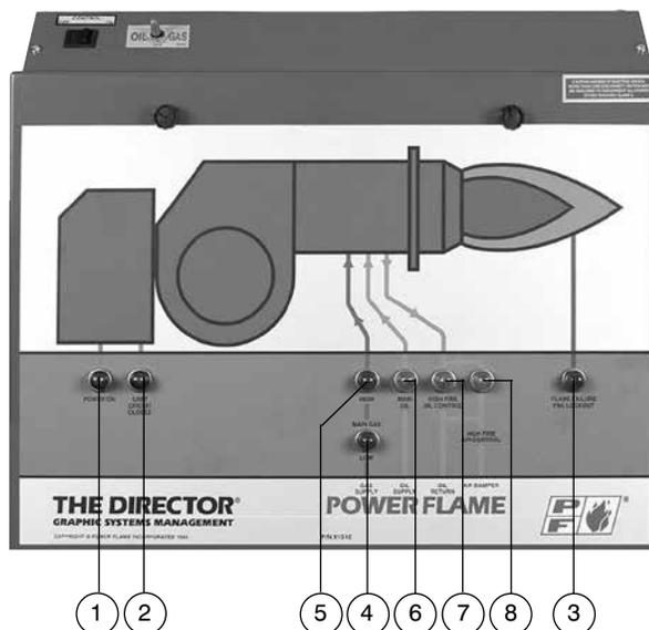
**Annunciation Legend for Gas/Oil Burner with Low-High-Low Operating Mode**
