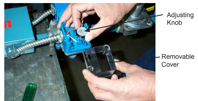
Figure E – 8 Gas Pressure Switch Adjustment
