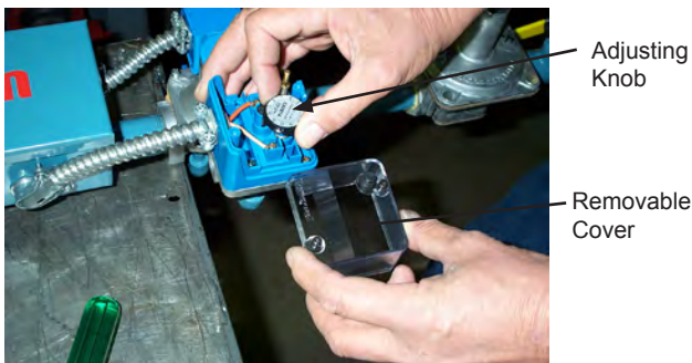
Figure E – 10 Gas Pressure Switch Adjustment
