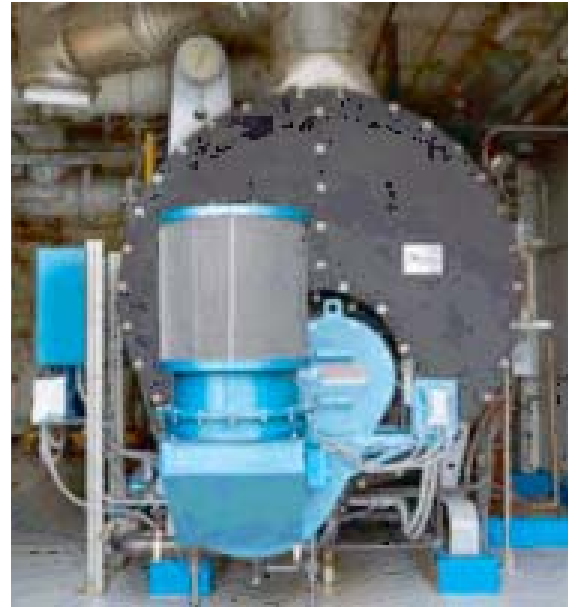
HDFX BURNER INSTALLATION
