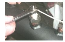
The high temperature wires attached to the probes can be routed to a local junction box or directly to the control unit. If a junction box is used, a low cost 18 Ga. Multi-conductor cable may be used to carry the signal to the control unit. We suggest Belden #8467 or equal.
